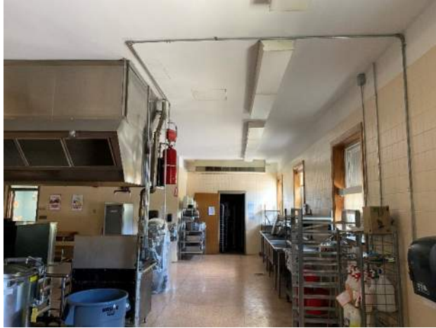
Image 11: Kitchen Unit Ventilator and Hood
