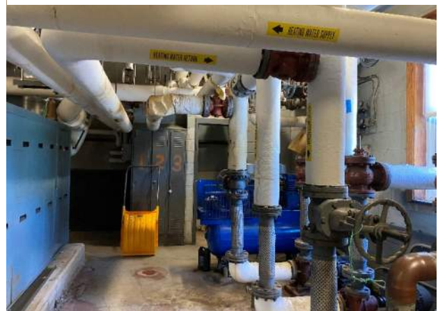
Image 4: Heating Hot Water Pipe Insulation with Water Damage
