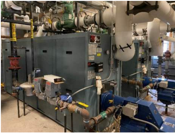
Image 1: HB Smith Cast Iron Boilers, Model 28HE-17
