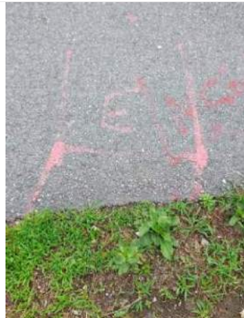
Dig Safe Electrical Ductbank Markings
