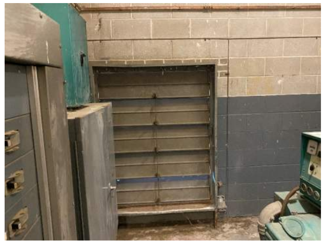
Image 18: Generator Room Make-up Air Louver
