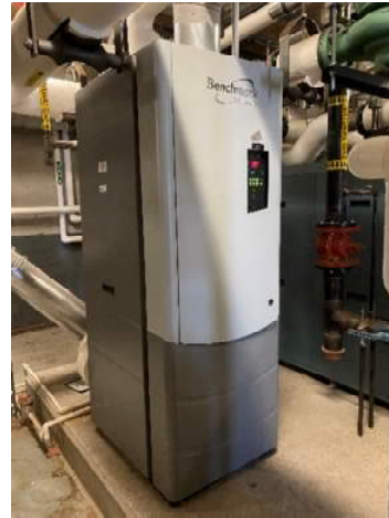
Image 2: Aerco gas-fired Condensing Boiler, Model Benchmark 2.0
