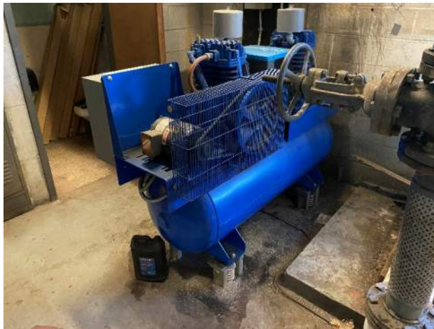
Image 5: Newer Quincy Pneumatic Controls Compressor
