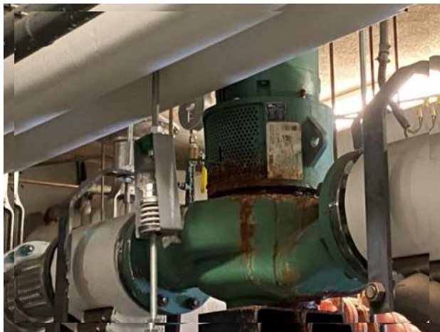
Image 3: Existing Boiler Pump With Signs of Leaking
