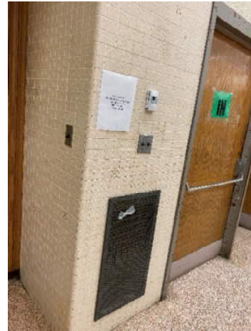
Image 14: Typical Low Wall Relief/Exhaust Grille
