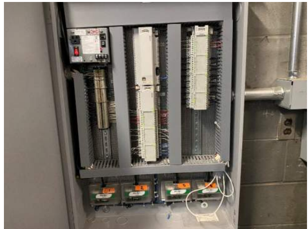
Image 6: Direct Digital Controls Cabinet in Mechanical Room
