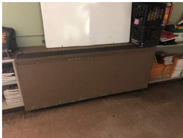
Image 1: Typical Classroom Unit Ventilator
