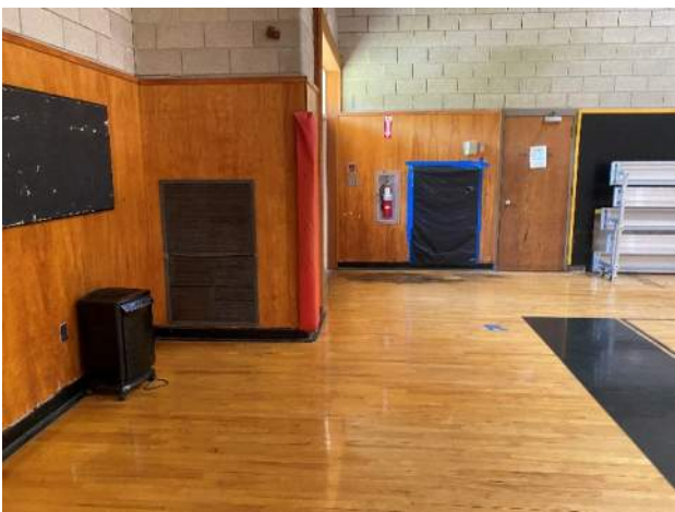
Image 10: Low Wall Exhaust/Relief Grilles (Note: Left Grille Damaged, Right Grille Covered/Blocked)
