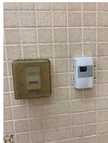
Image 16: Old Pneumatic, and New DDC Thermostats
