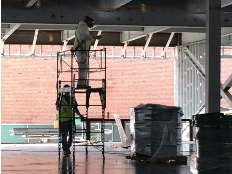
SPRAY FIREPROOFING 2ND FLOOR AREA A
