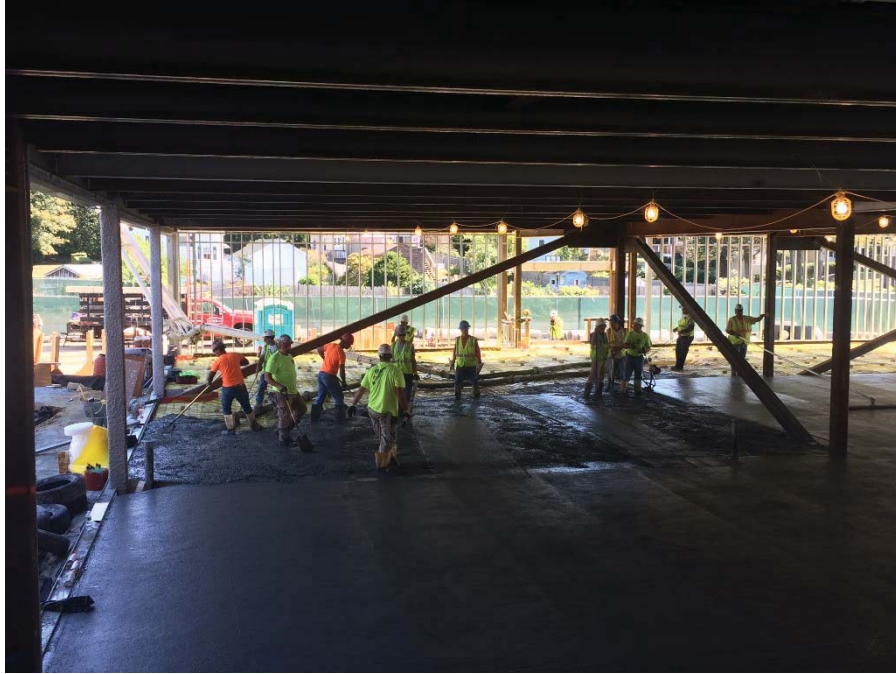
PLACING 3RD FLOOR SLAB AREA A
