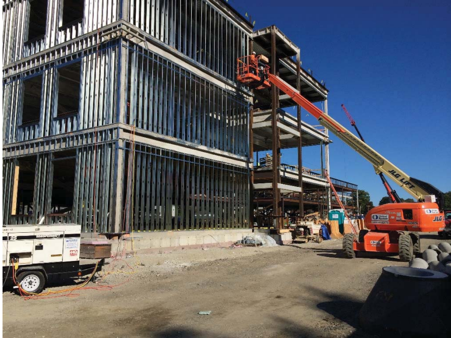
EXTERIOR LIGHT GAGE METAL FRAMING EAST WALL AREA A
