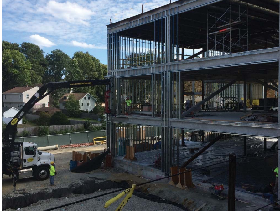
EXTERIOR LIGHT GAGE METAL FRAMING AREA A
