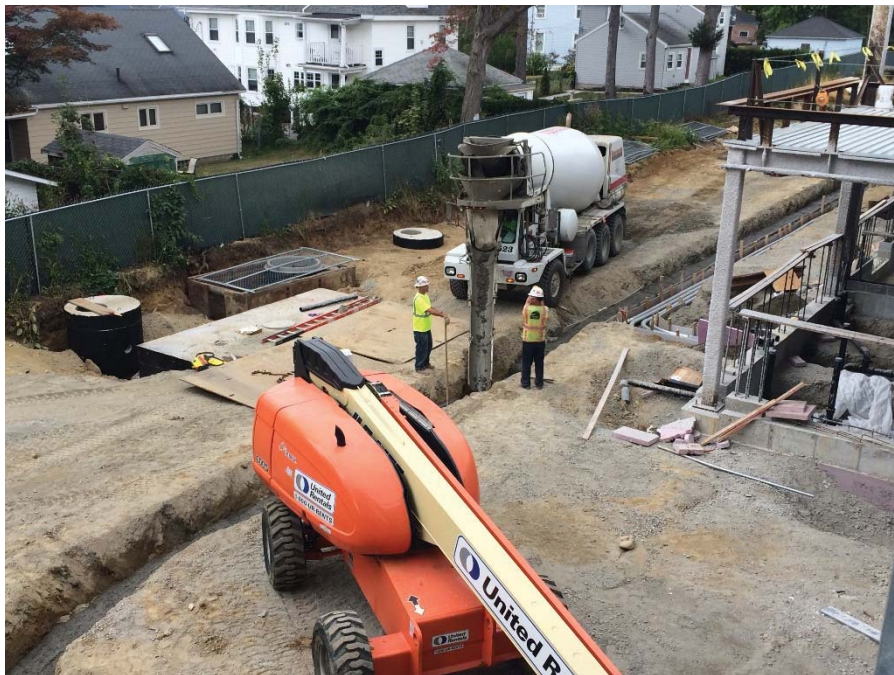
POURING CONCRETE ENCASED ELECTRICAL AND DATA DUCT BANK
