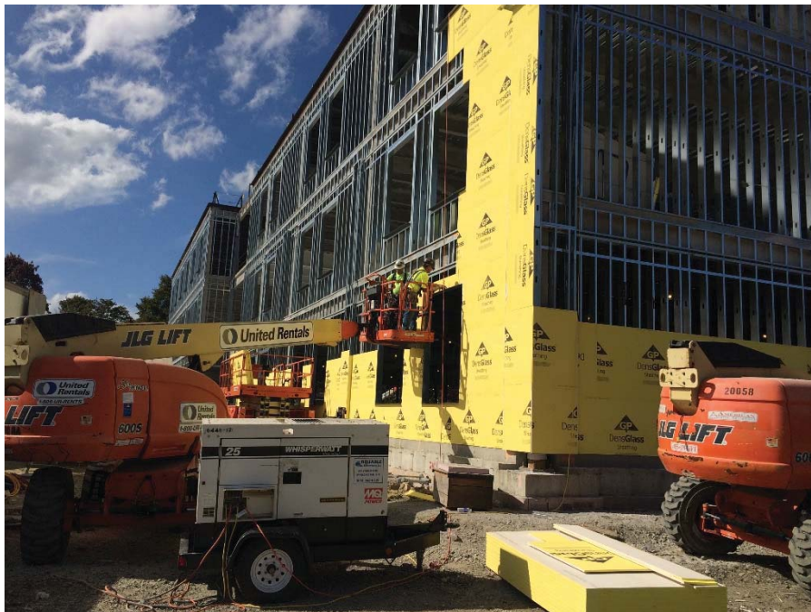
EXTERIOR SHEATHING SOUTH EAST CORNER OF AREA A
