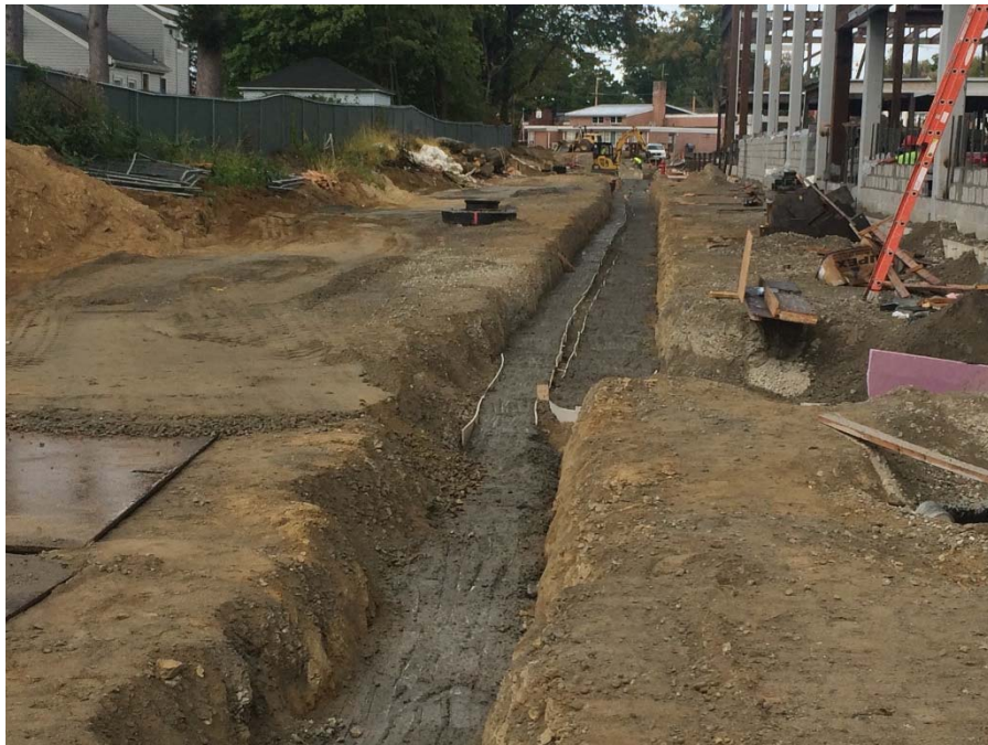
ELECTRICAL DUCT BANK
