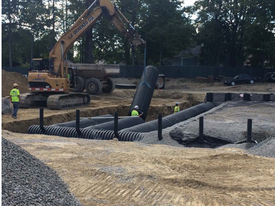
UNDERGROUND RETENTION SYSTEM
