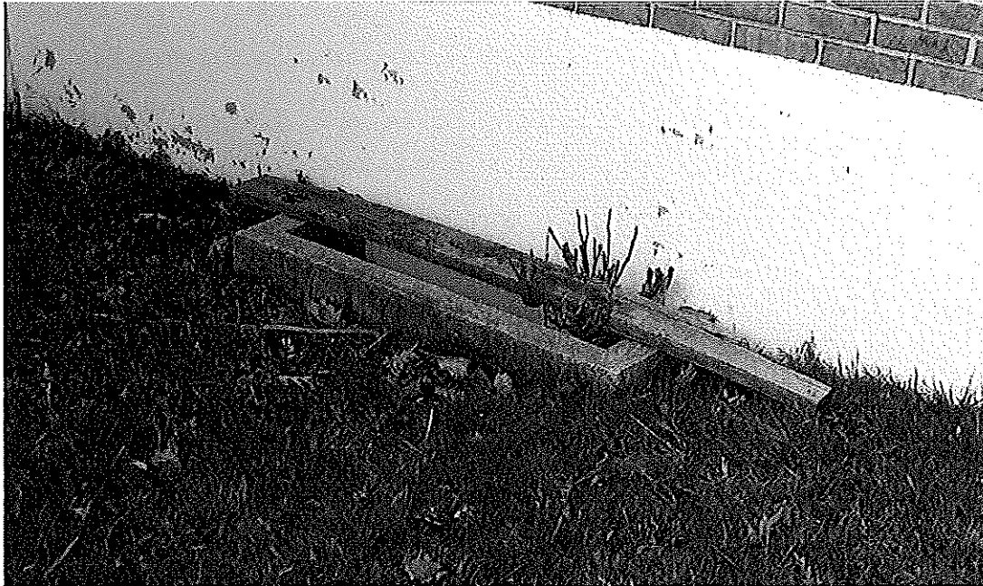
Sealed crawlspace vent near building entrance
