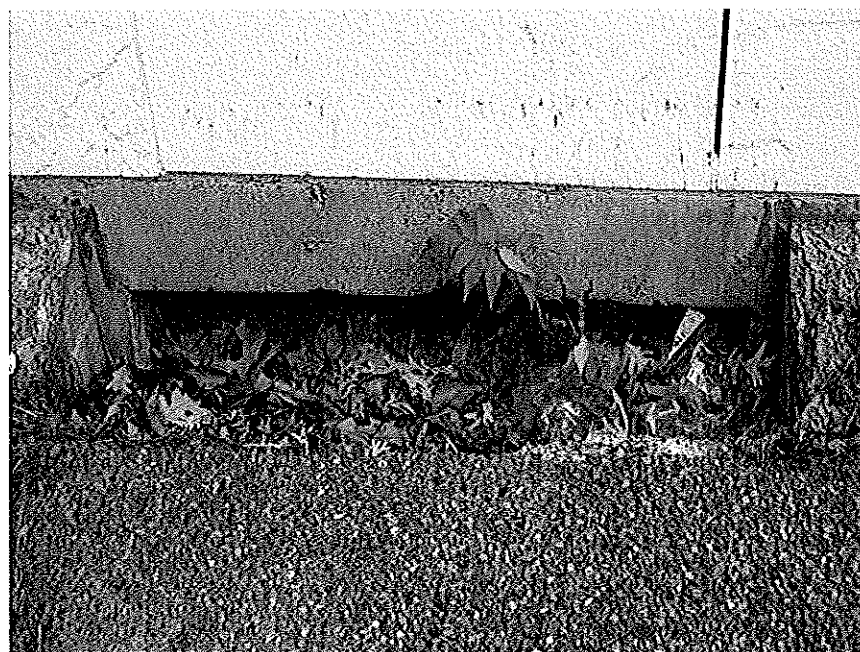
Sealed crawlspace vent near gymnasium
