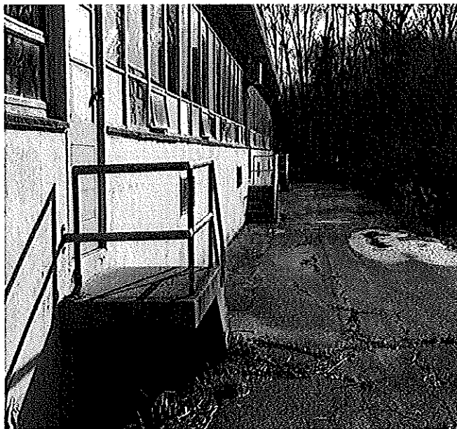
Crawlspace exhaust vents below staircases, note orientation of staircase 1 (foreground) and staircases 2 and 3 (background)
