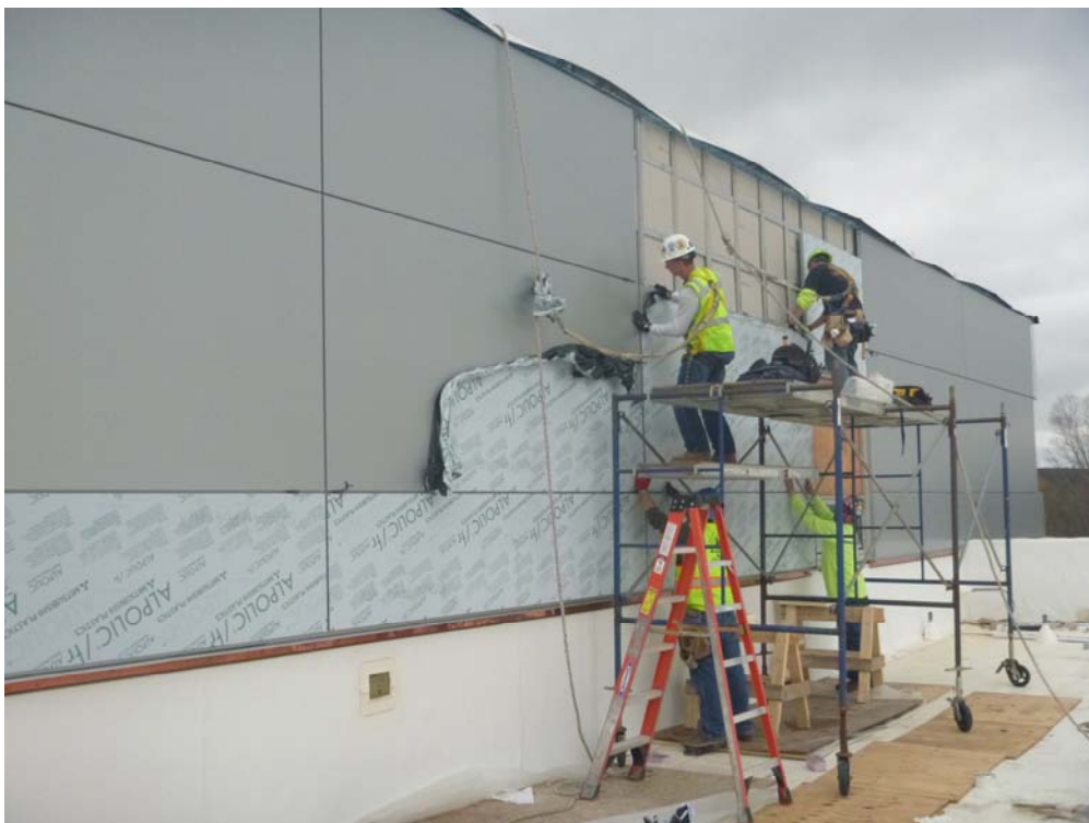
PREFINISHED METAL PANEL INSTALLATION NORTH FACADE AREA A
