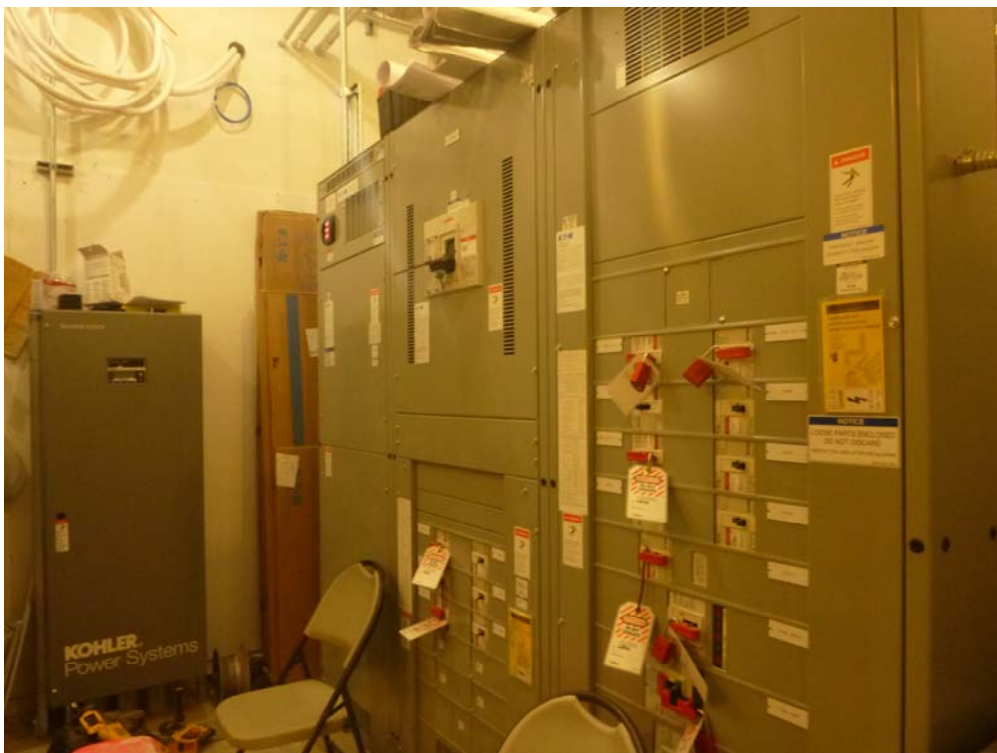
MAIN SWITCHGEAR ENERGIZED
