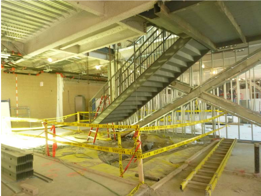
STEEL STAIR FRAMING AND RAILINGS INSTALLED
