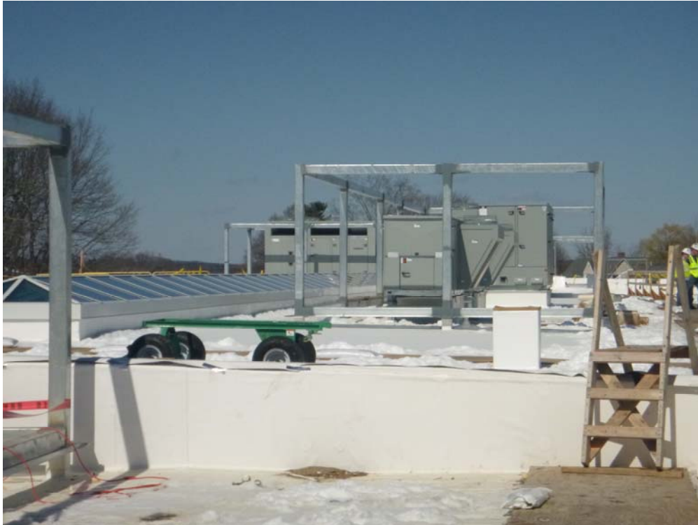
MECHANICAL ROOFTOP UNITS DELIVERED AND PLACED ON CURBS
